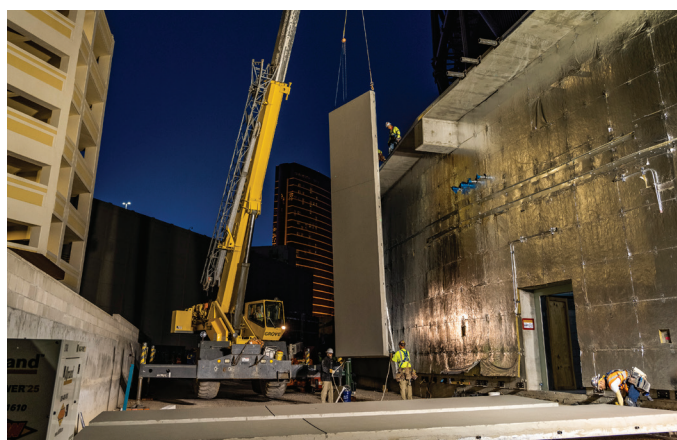
Outsulite panel installation
